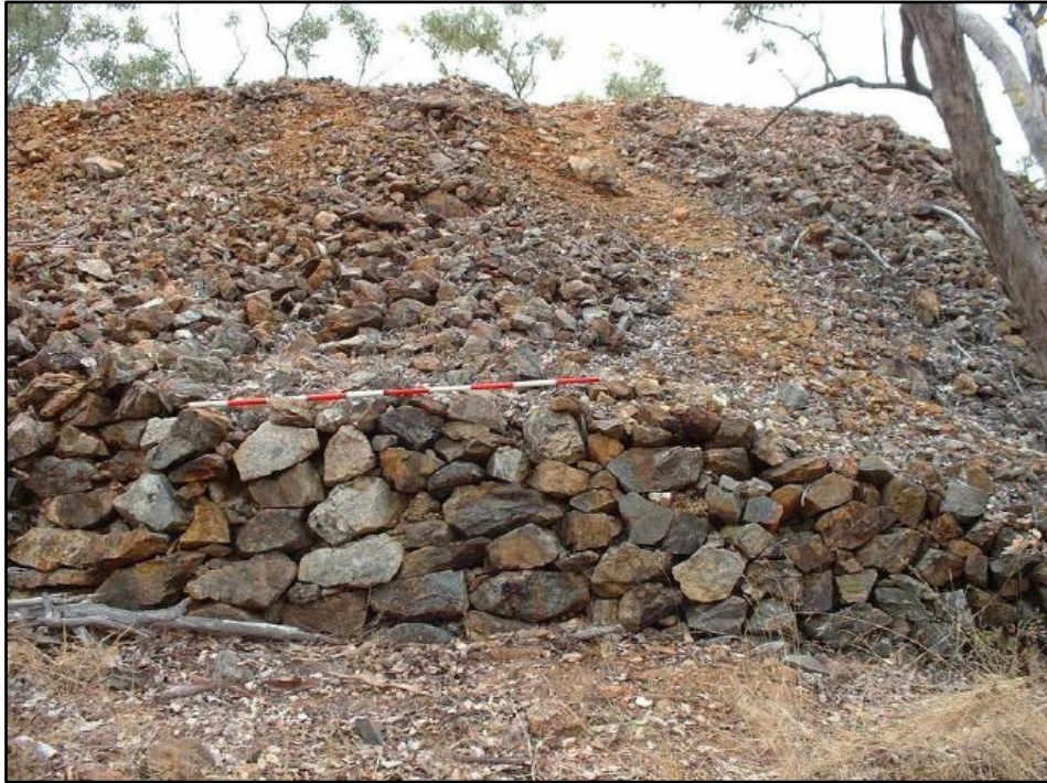
Figure 17: The Mowbray Mine's mullock heap with drystone retaining wall (Taylor 2005 in Taylor 2013)
