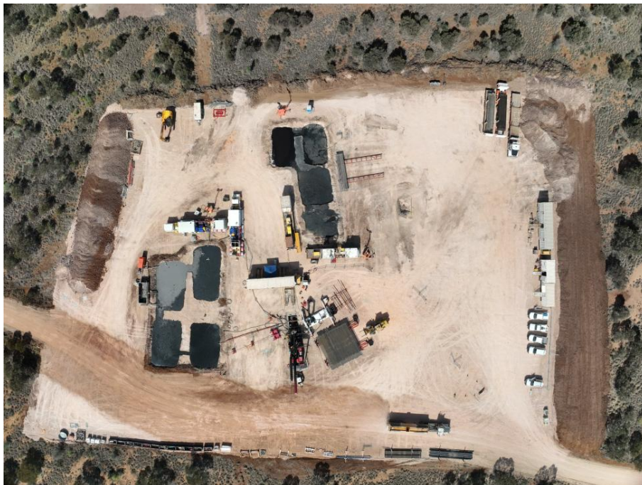
Image 2.2 Example of drill pad arrangement
