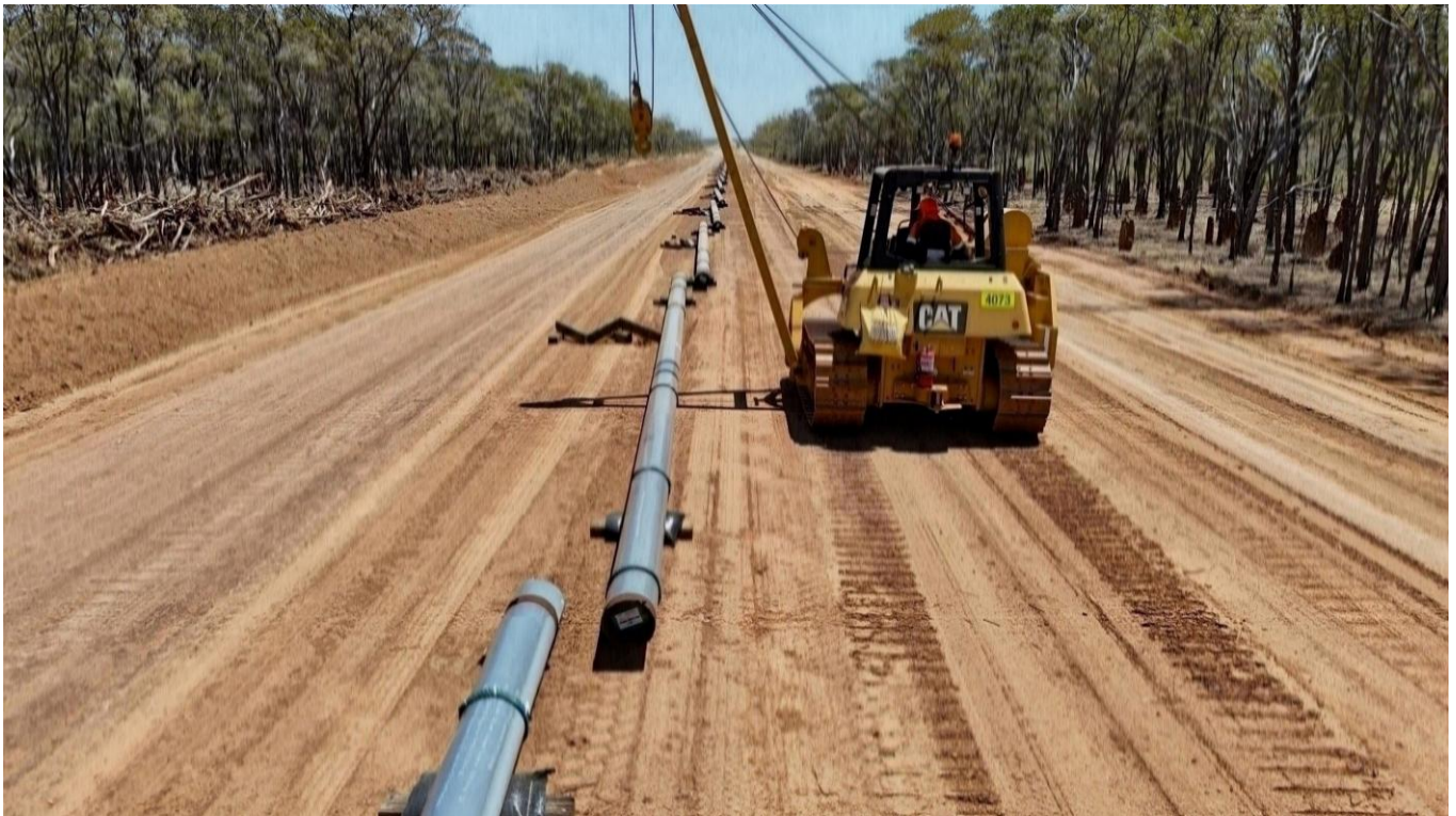
Plate 4.2 Example of pipeline stringing (source: APA 2026)
