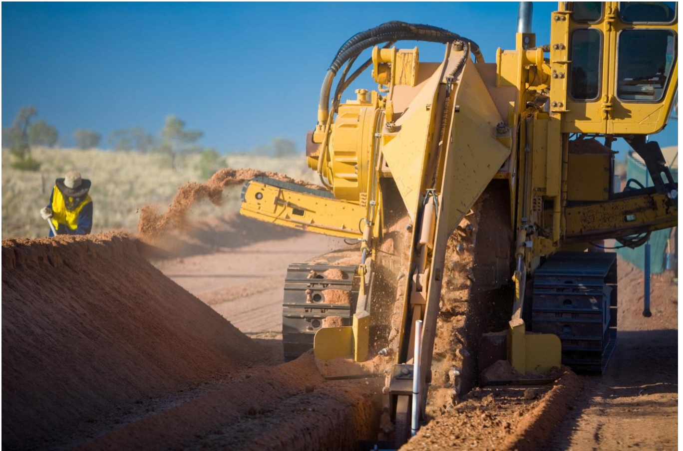
Plate 4.3 Example of open trenching and spoil placement (source: APA 2026)
